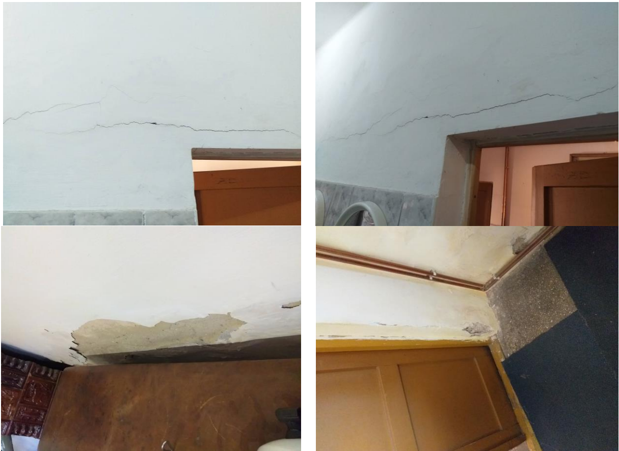
Figure 5. Current state of the buildings, windows, doors, heating system (wood stove)
